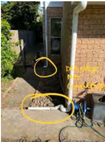
No Down Pipe Ground Connections
