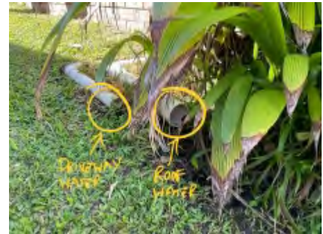
There is no in-ground drainage reticulation to take roof water away from the property.
