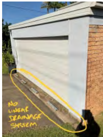
The drain to the front of the garage appears to be undersized to cope with surface water. Additionally there is no connection to an in ground drainage reticulation system to take water out to the street.
