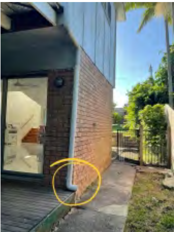
No Down Pipe Ground Connections
