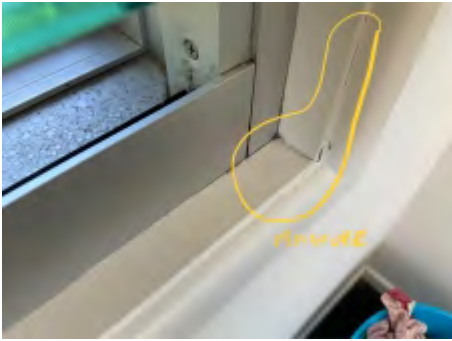
Many of the windows appear to be letting water. Signs of cracking and moisture damage to architraves generally throughout.
