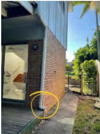
There is no in-ground drainage reticulation to take roof water away from the property.
