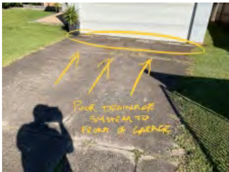
The drain to the front of the garage appears to be undersized to cope with surface water. Additionally there is no connection to an in ground drainage reticulation system to take water out to the street.
