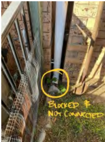
No Down Pipe Ground Connections
