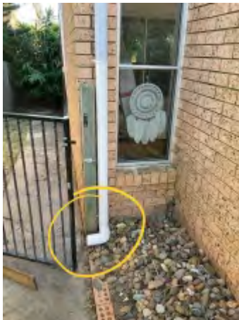
No Down Pipe Ground Connections
