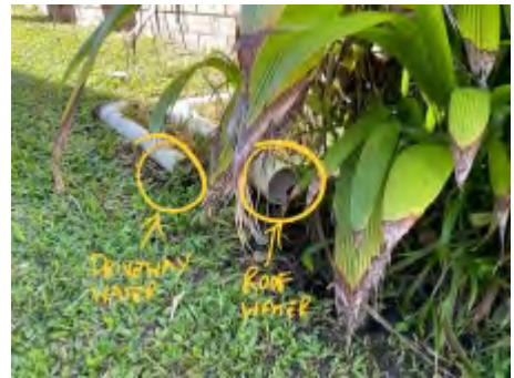
No Down Pipe Ground Connections
